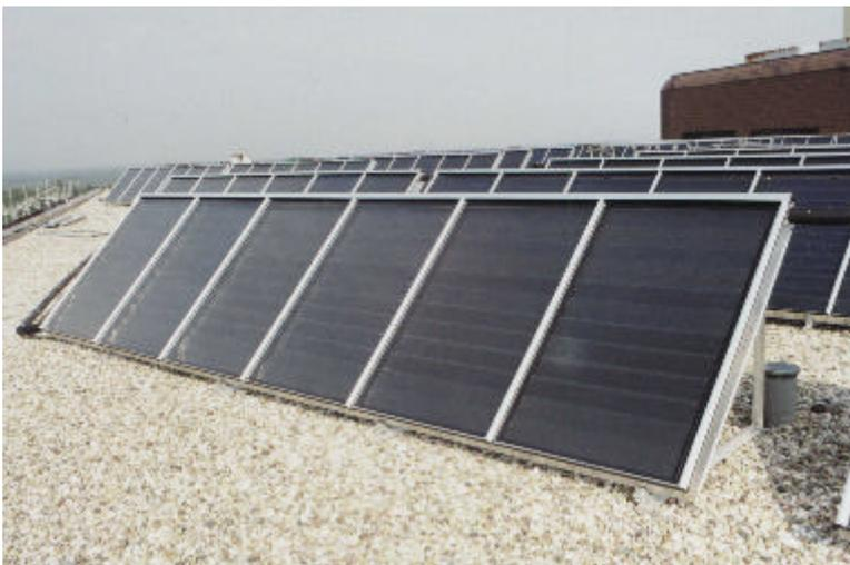
Fig. 1: Flat plate collectors of the solar thermal plant in the hospital in Baden-Baden
